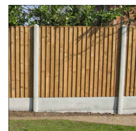
Panel fence with concrete post and gravel boards
